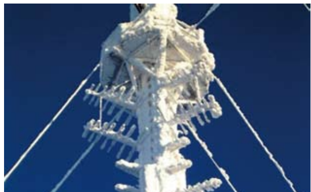
An ice covered Huawei base station in the Arctic Circle area of Finland.
